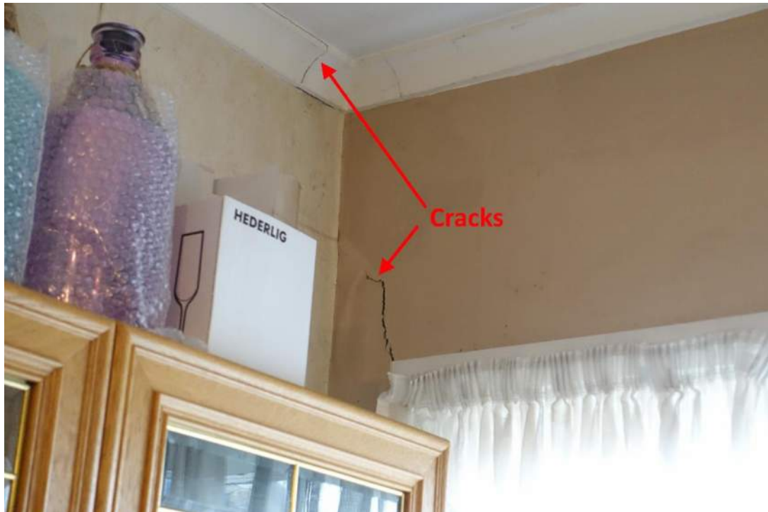
Photograph 46: Wall and ceiling cracking at first floor
