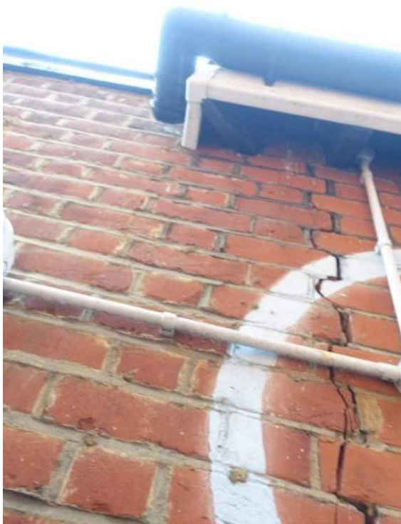
Photograph 32: Severe cracking in the north flank wall
