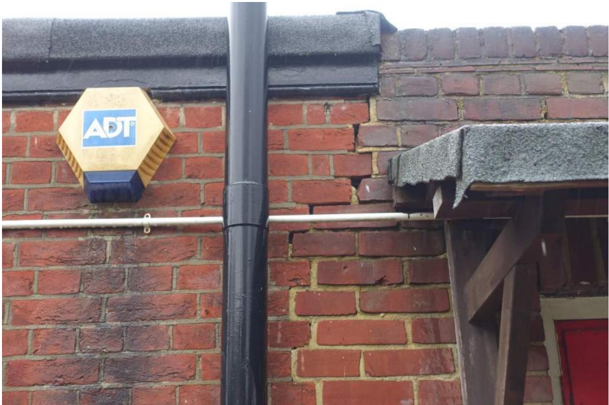
Photograph 10: Cracking and open joints on the west elevation
