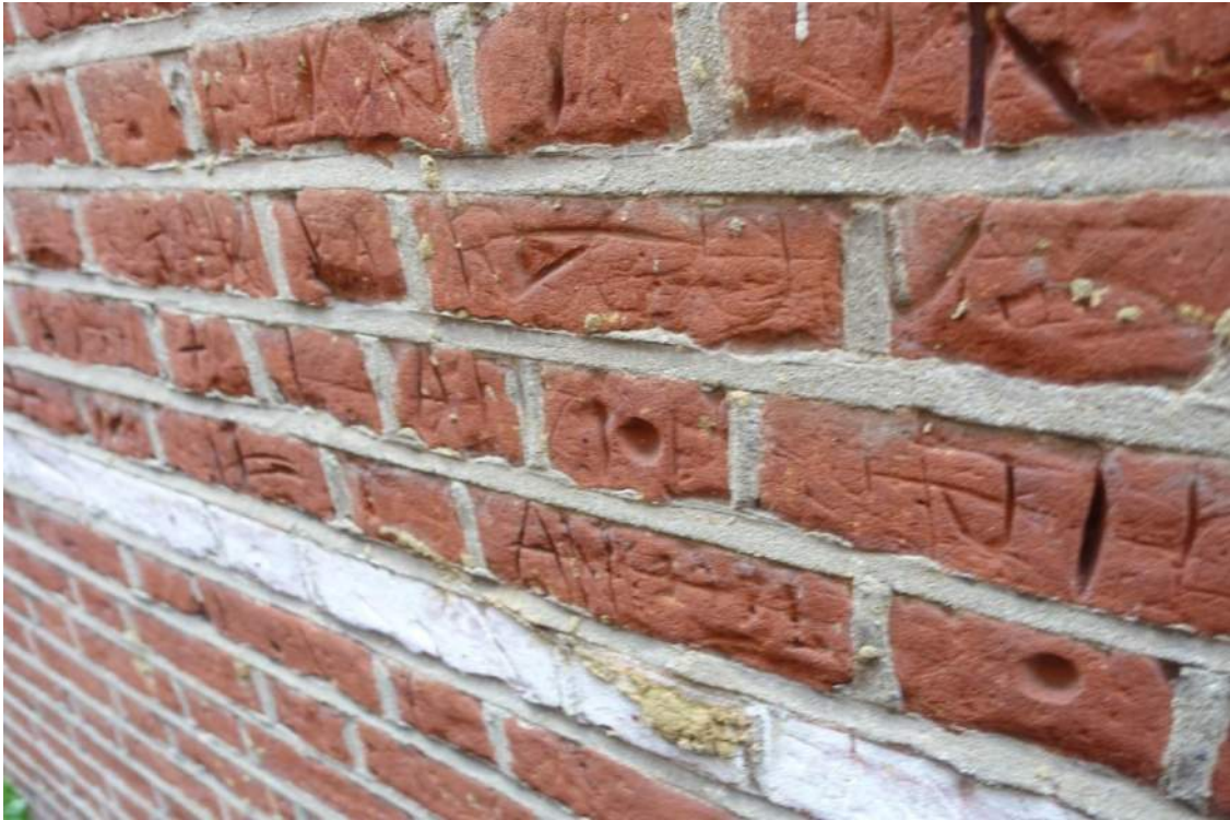
Photograph 35: Damage to the brickwork surface by vandals
