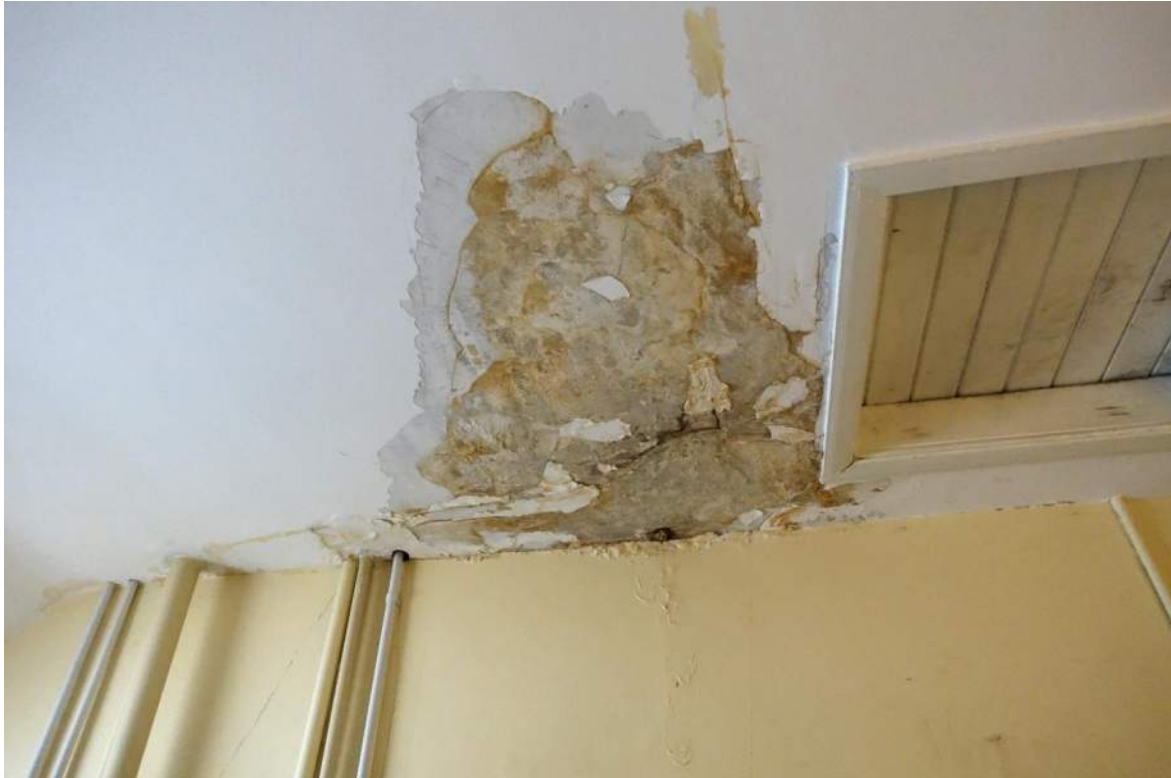
Photograph 22: Apparent damp damage in the ceiling over a first floor office
