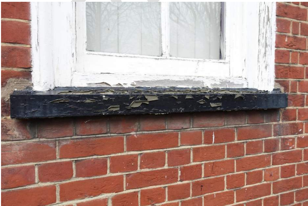
Photograph 15: Flaking/missing paint on window frames and cills
