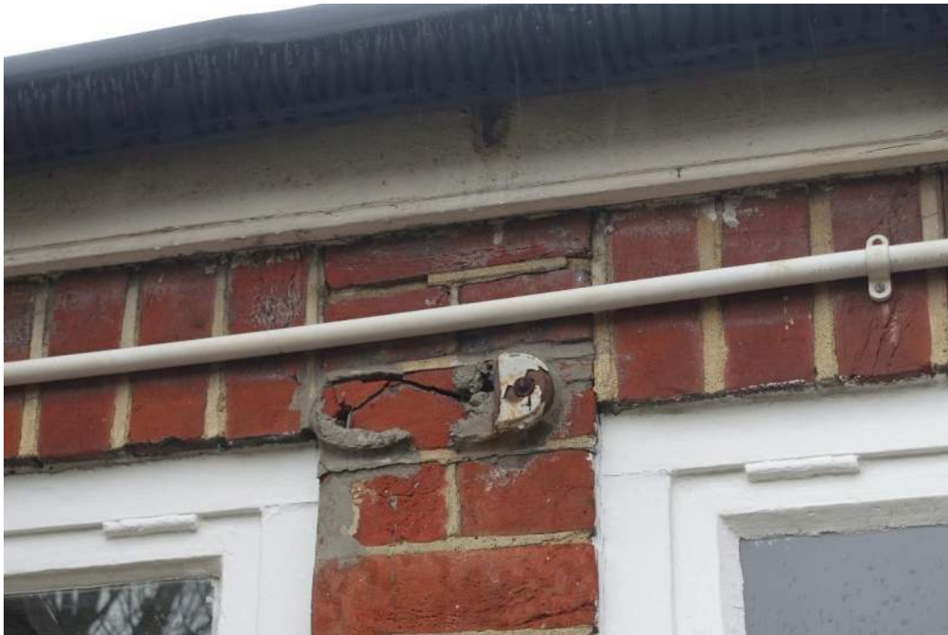
Photograph 12: Damaged brickwork at a redundant fitting
