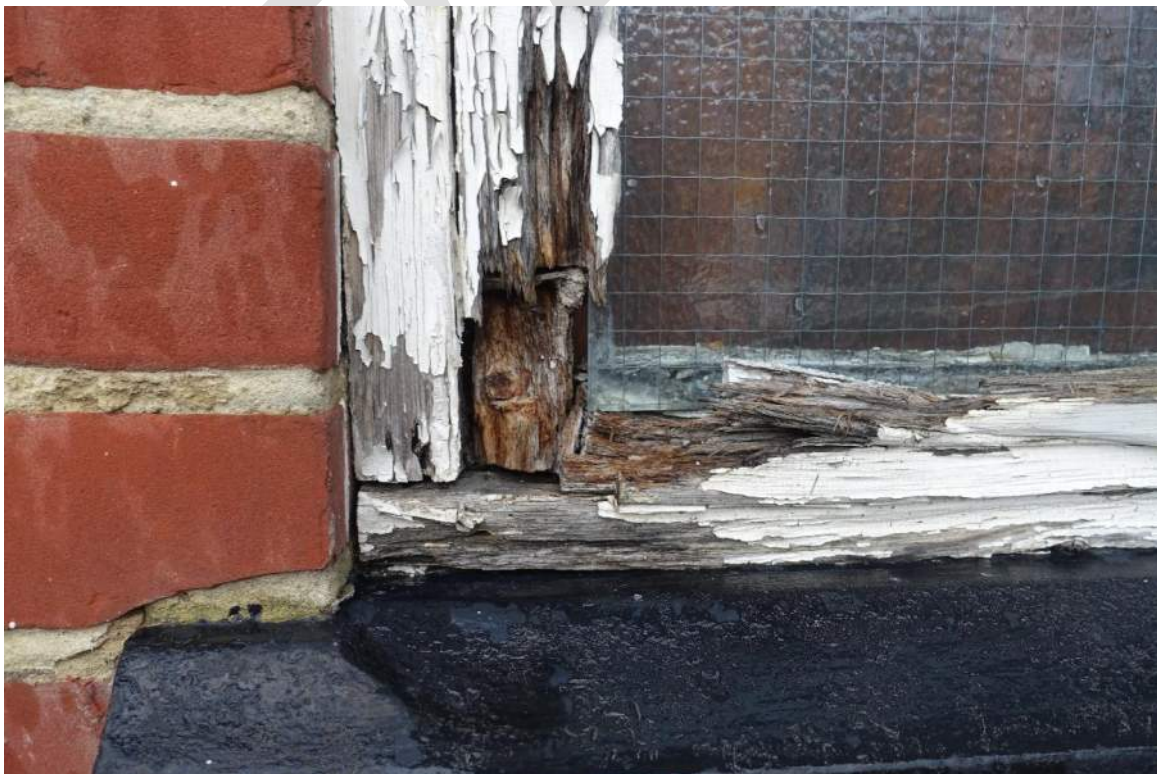
Photograph 17: Rotten window frame timbers
