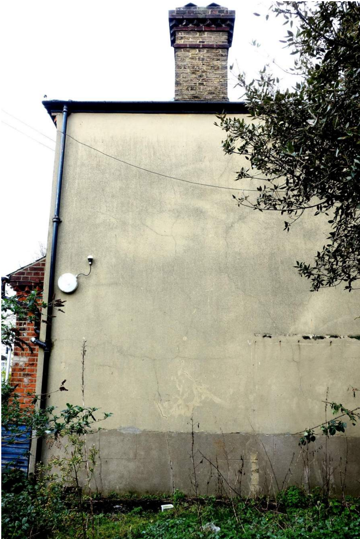
Photograph 39: Cracked rendered flank wall
