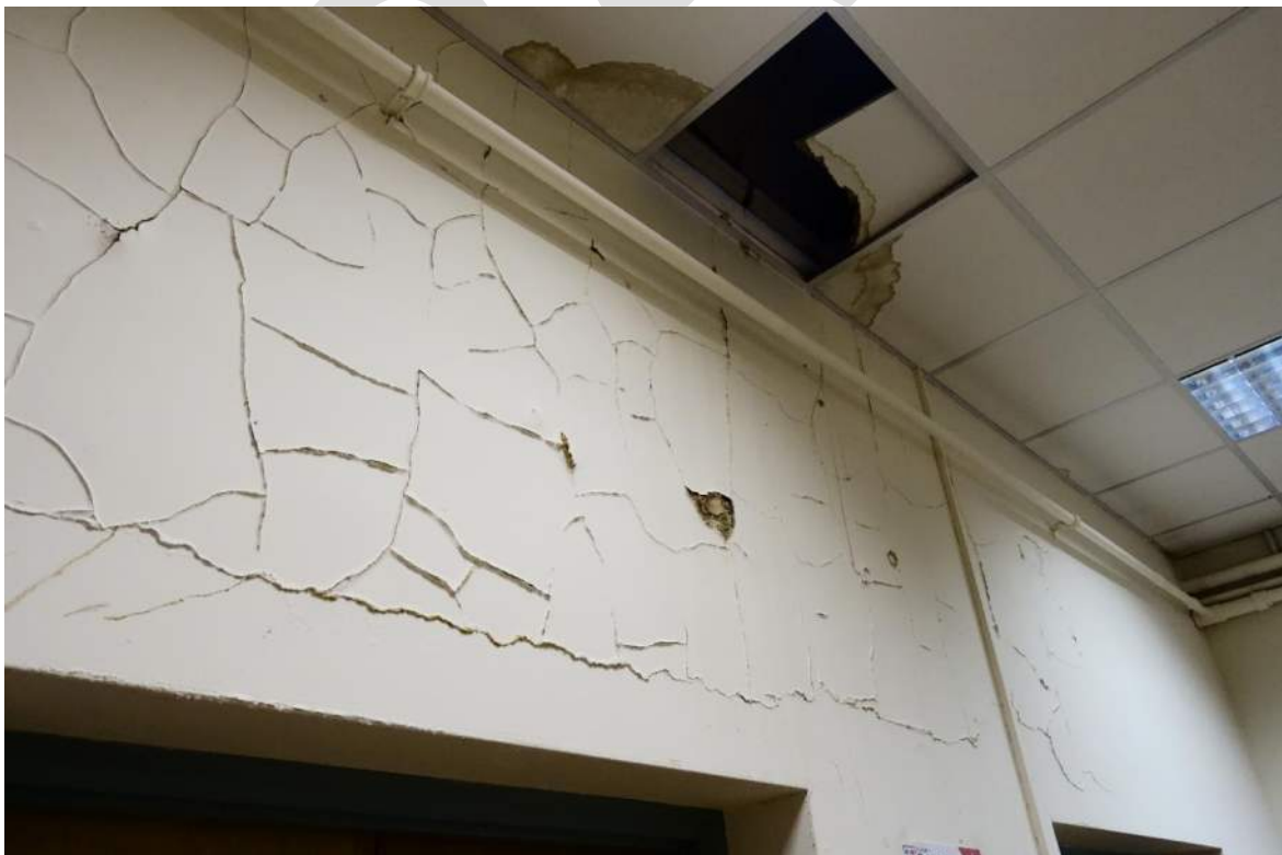
Photograph 23: Evidence of damp in the ceiling of a ground floor multifunction room
