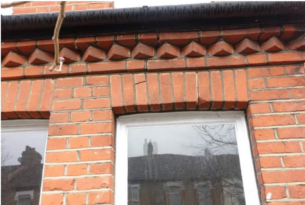
Photograph 30: Cracked brickwork at an arch
