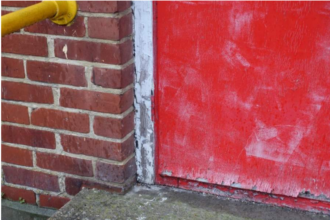
Photograph 16: Missing/flaking paint to door frame and door. The timber door is delaminating Some window frame timbers are badly rotting.
