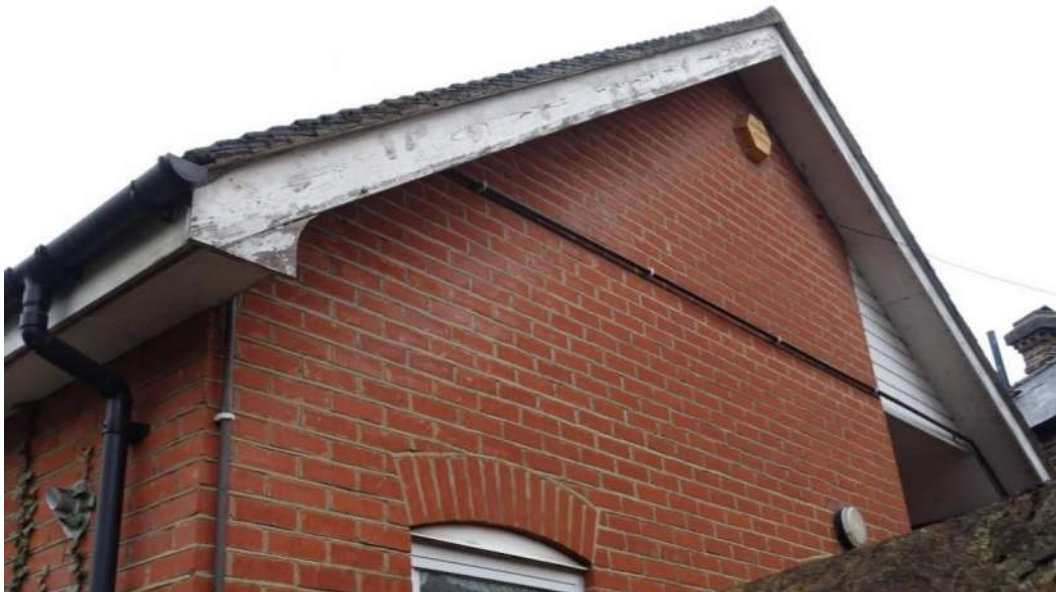
Photograph 28: Barge boards need repainting
