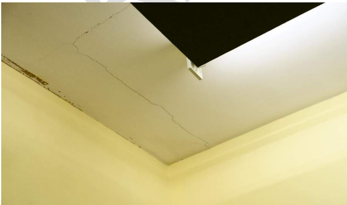
Photograph 27: Minor ceiling cracking
