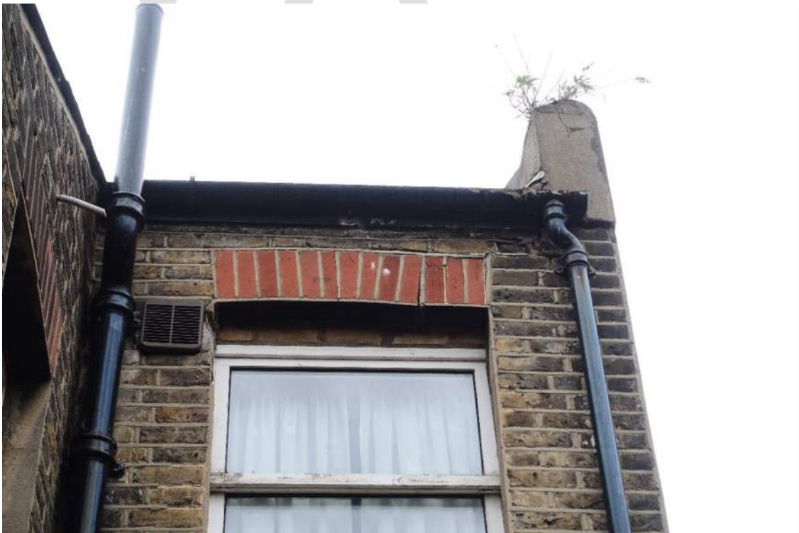
Photograph 36: A deformed and cracked brick arch over a window
