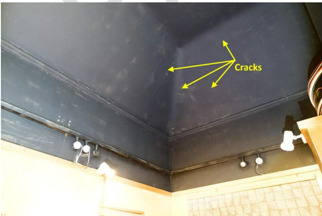
Photograph 21: Cracking in bar ceiling
