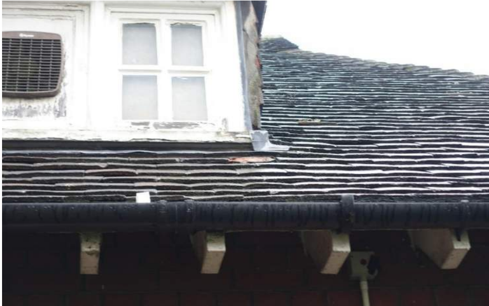
Photograph 18: Poor condition paintwork on dormer window. Roof tiling appears to be breaking up Reportedly, the felt roof over the eastern plantroom and store was replaced about 8 years ago.
