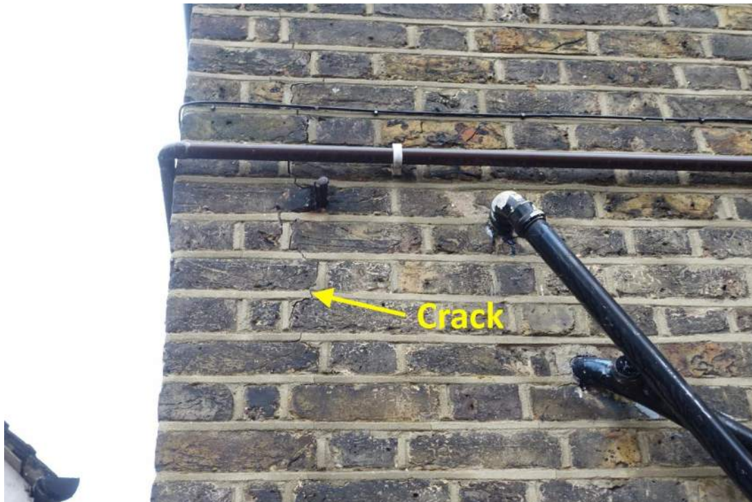
Photograph 37: Cracking in a repointed wall
