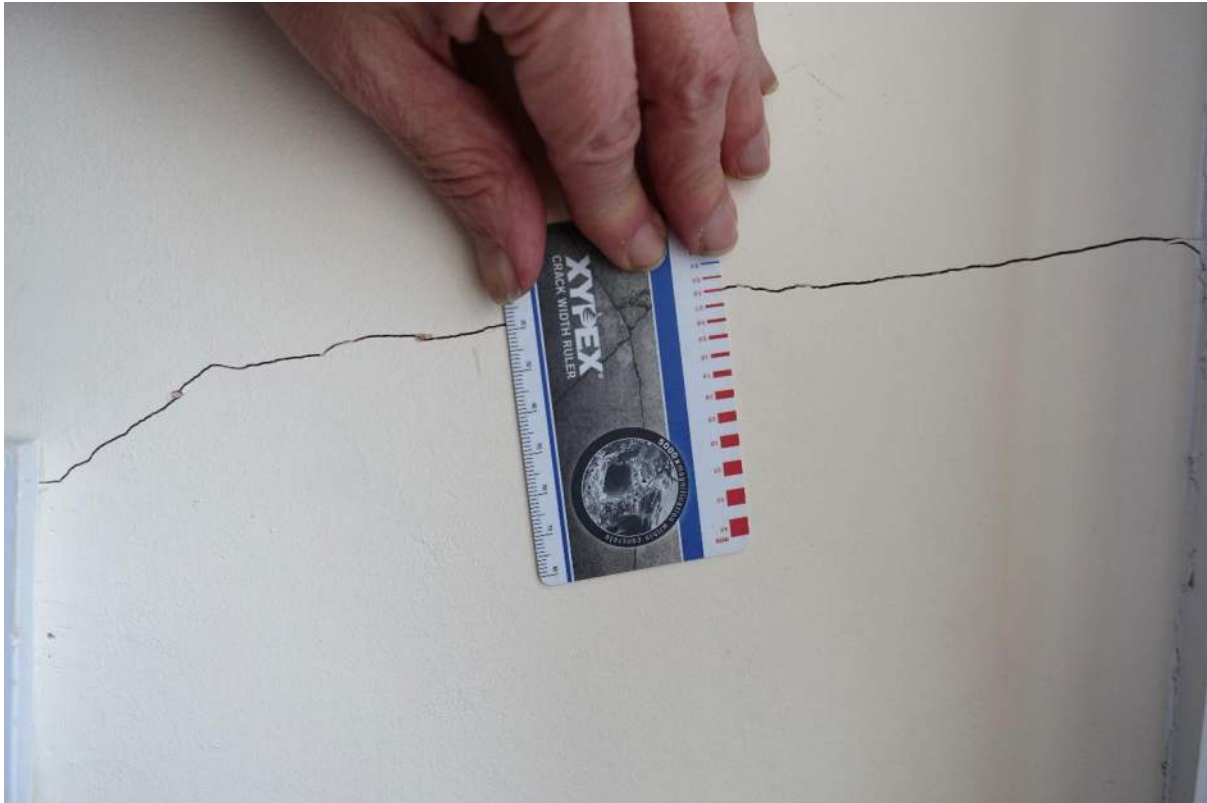
Photograph 42: A wall crack measured at 0.6mm wide
