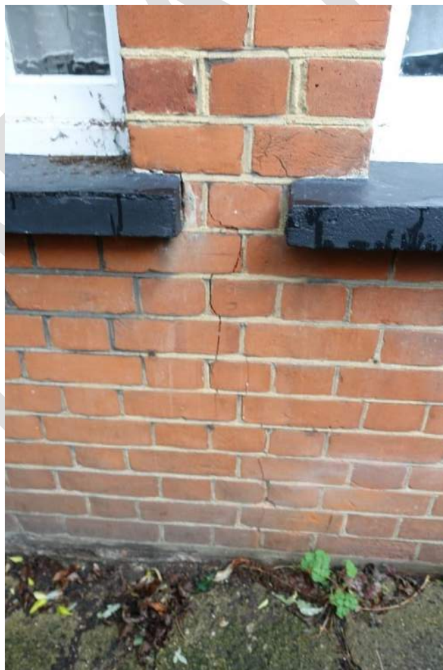
Photograph 31: Cracking, approximately 2mm wide, at the front
