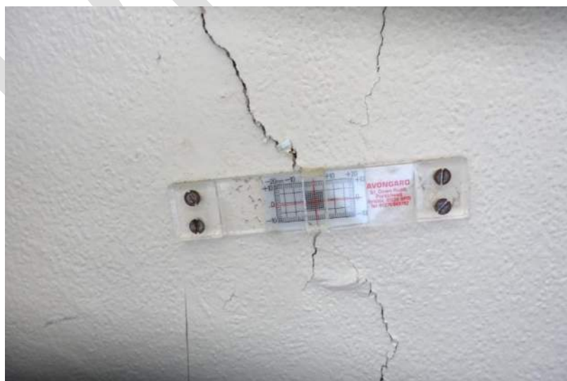
Photograph 29: Crack 'tell-tales' provide evidence of historical monitoring of the building's movement
