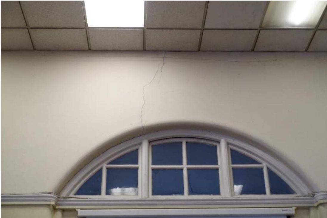
Photograph 20: Cracked arch in main hall
