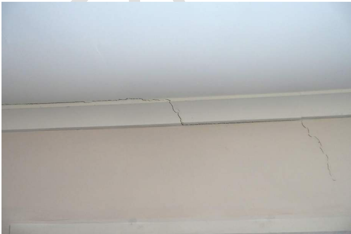
Photograph 45: Wall and ceiling cracking at first floor
