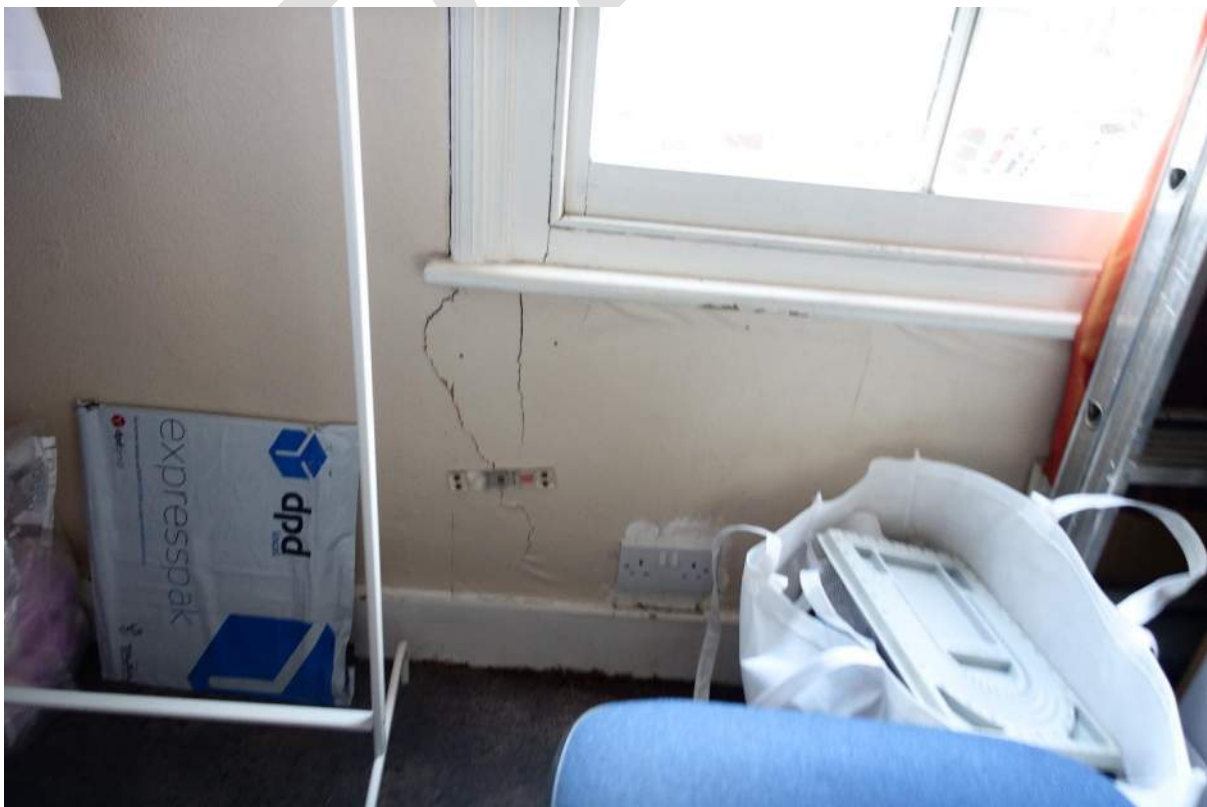
Photograph 43: 2mm wide cracking below a first-floor window.
