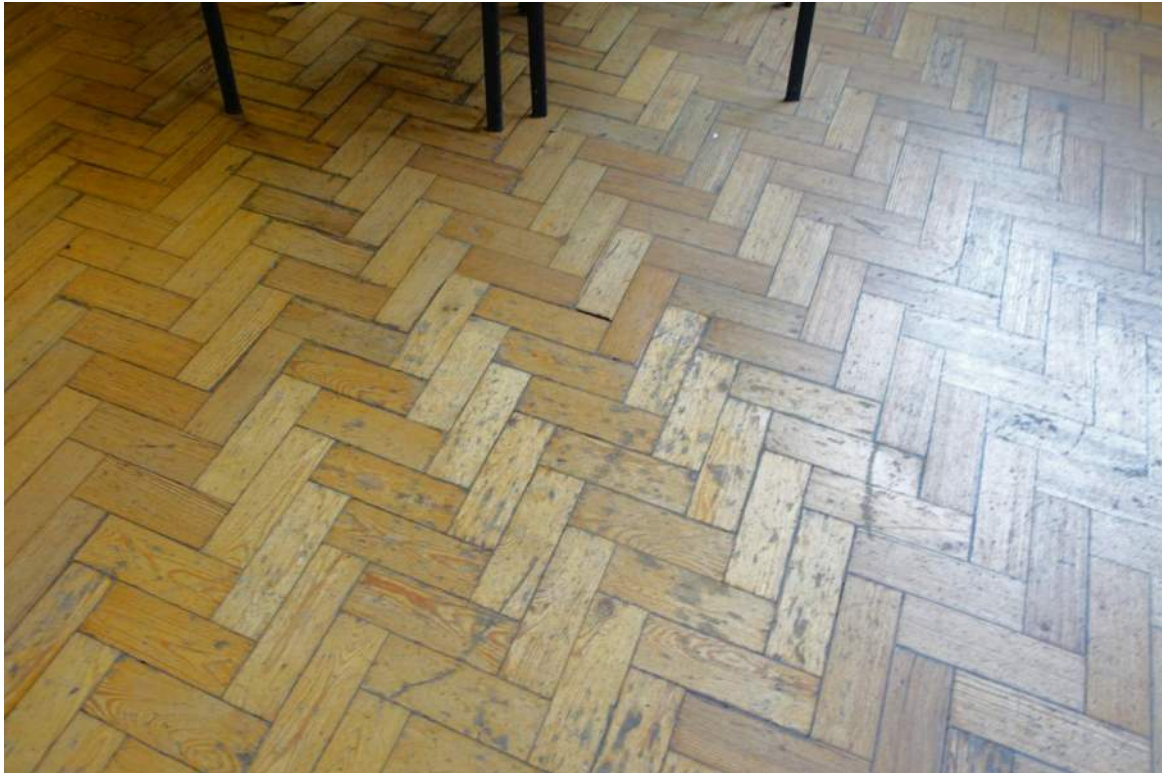
Photograph 26: Worn timber parquet floor in the main hall
