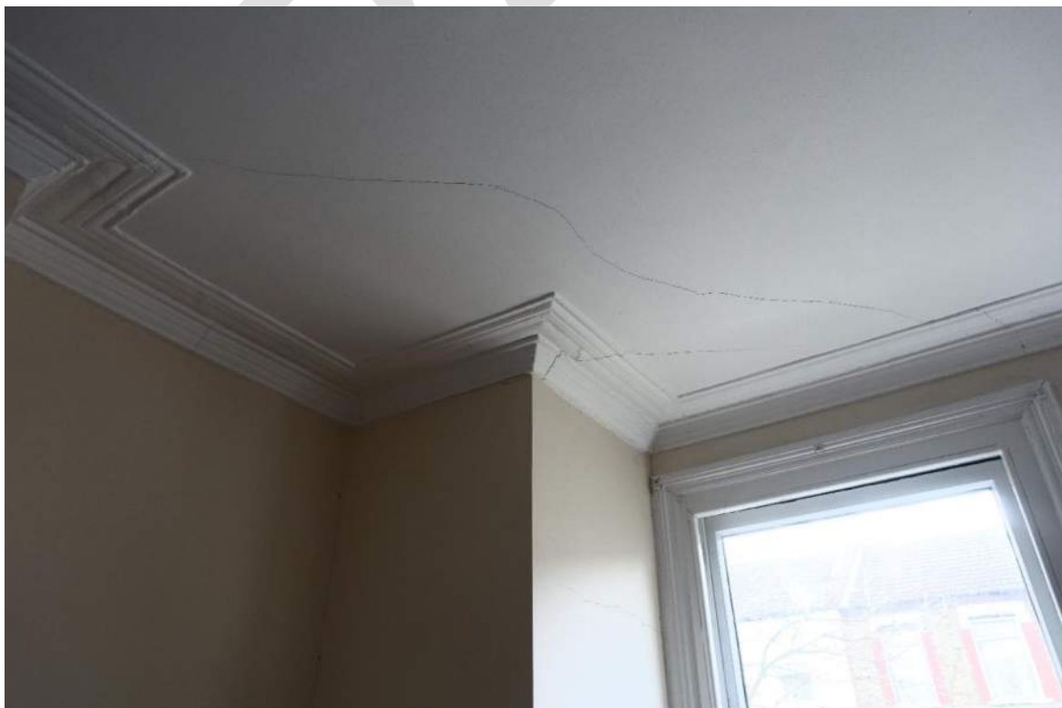
Photograph 41: Cracked ceiling at ground floor
