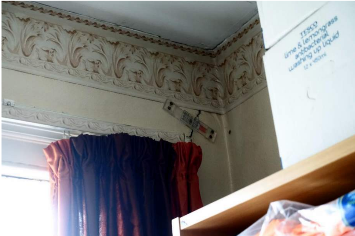
Photograph 44: Cracking above the window, with a tell-tale in place
