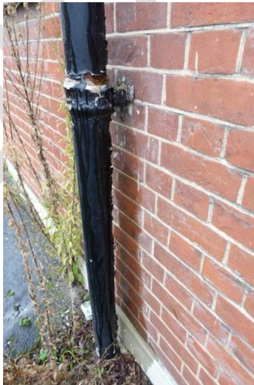
Photograph 19: Leaking/rusting rainwater downpipe
