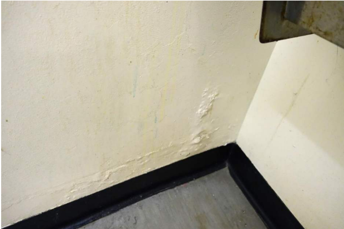
Photograph 24: Paint blistering within the Gentlemen's toilet may be due to damp
