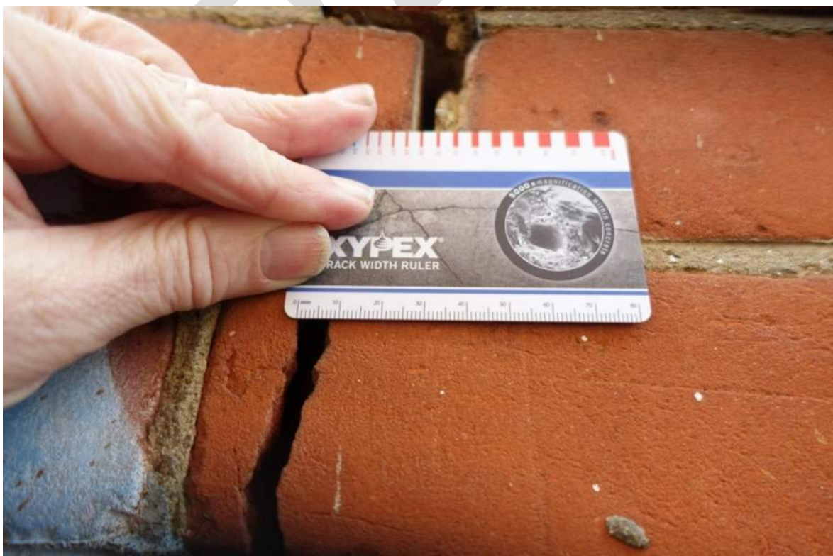
Photograph 34: The crack is 8mm wide at head height, widening to about 10mm higher up
