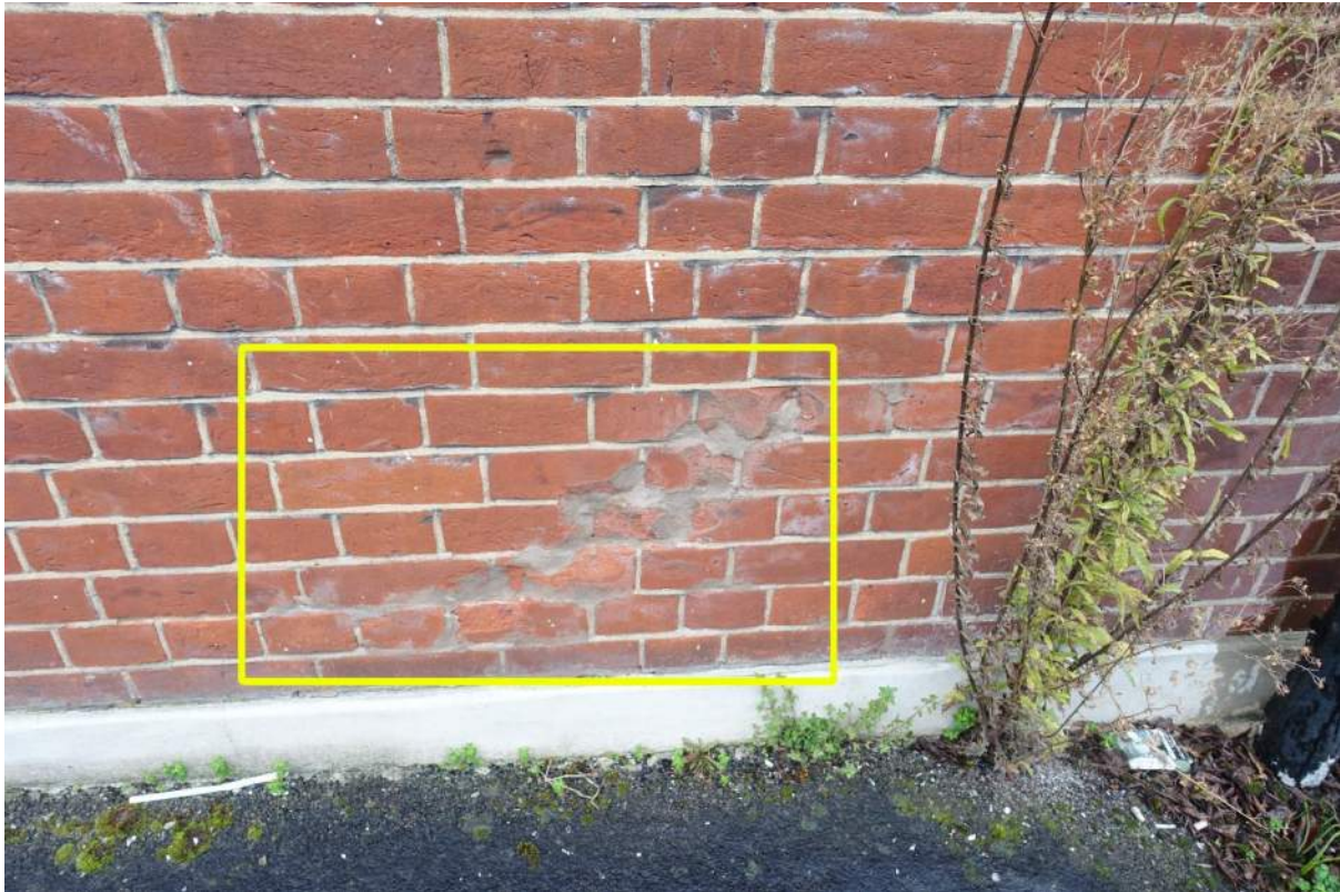
Photograph 14: Mortar repairs to spalled brickwork
