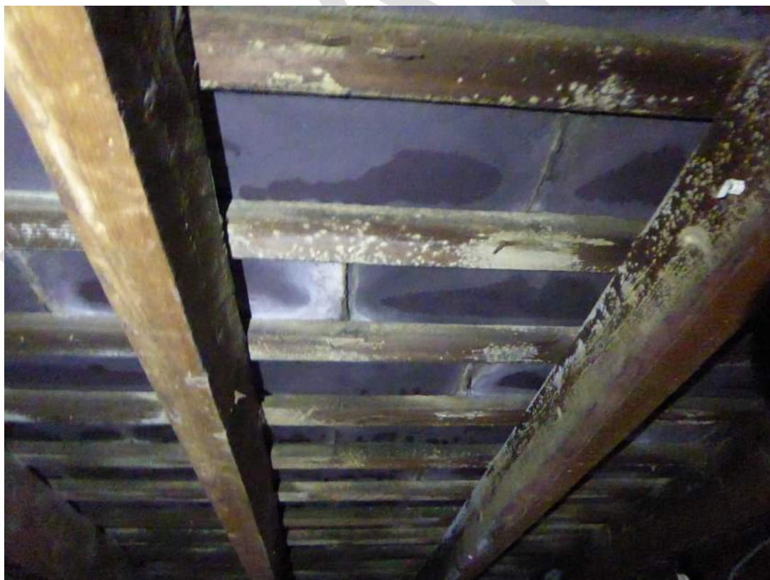
Photograph 47: Signs of damp within the roof space of Emily Villa
