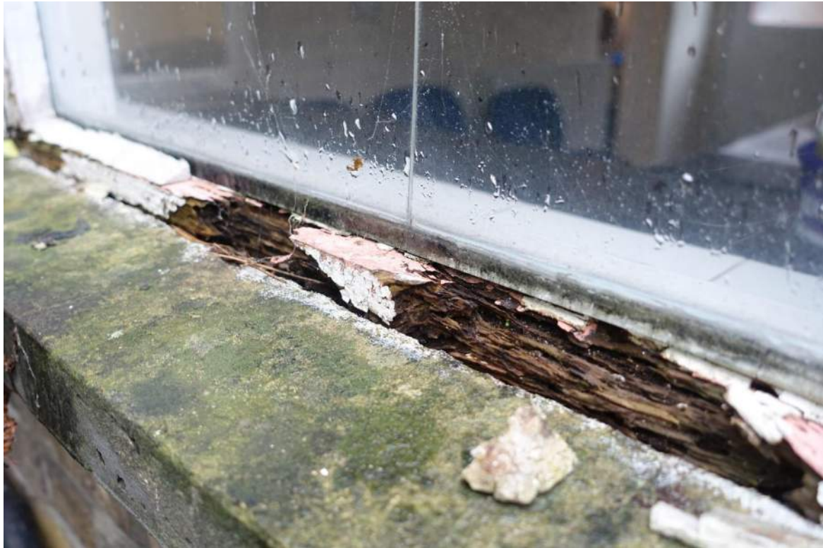
Photograph 40: Rotten timber to the rear
